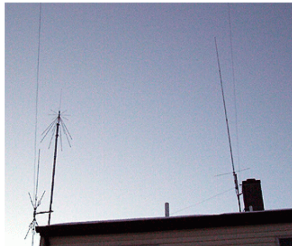
Roof Mounted Antennas
