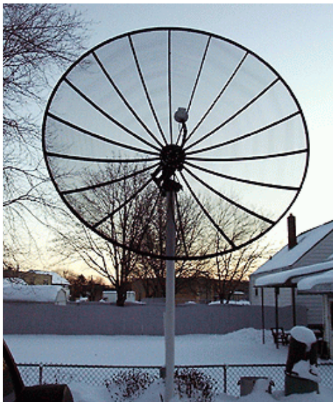
C / Ku Band Sat Dish
