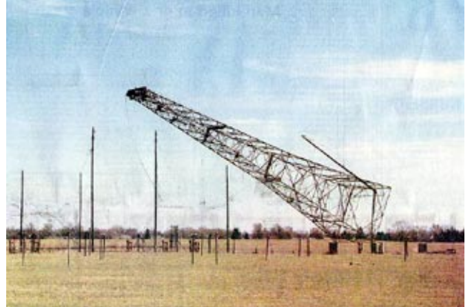
VOA TOWER COMING DOWN !
