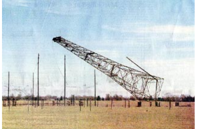
VOA TOWER COMING DOWN !
