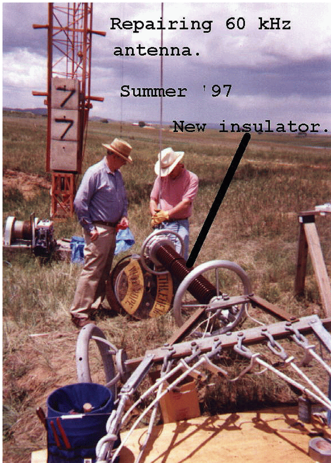
WWVB Insulator Repair
